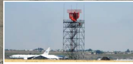
Airport Surveillance Radar (ASR)
