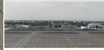
Terminal Area View from ATCT
